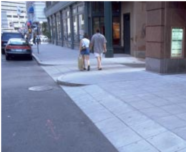
Driveway design integrated with sidewalk
