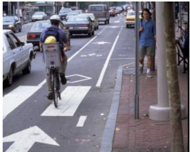
Example of bicycle pavement markings
