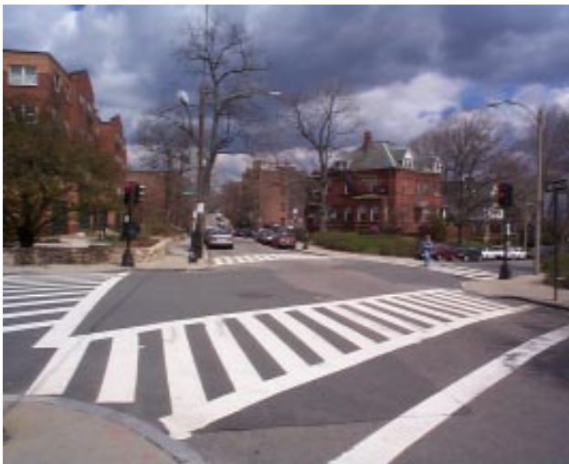
Crosswalks on all sides of an intersection
